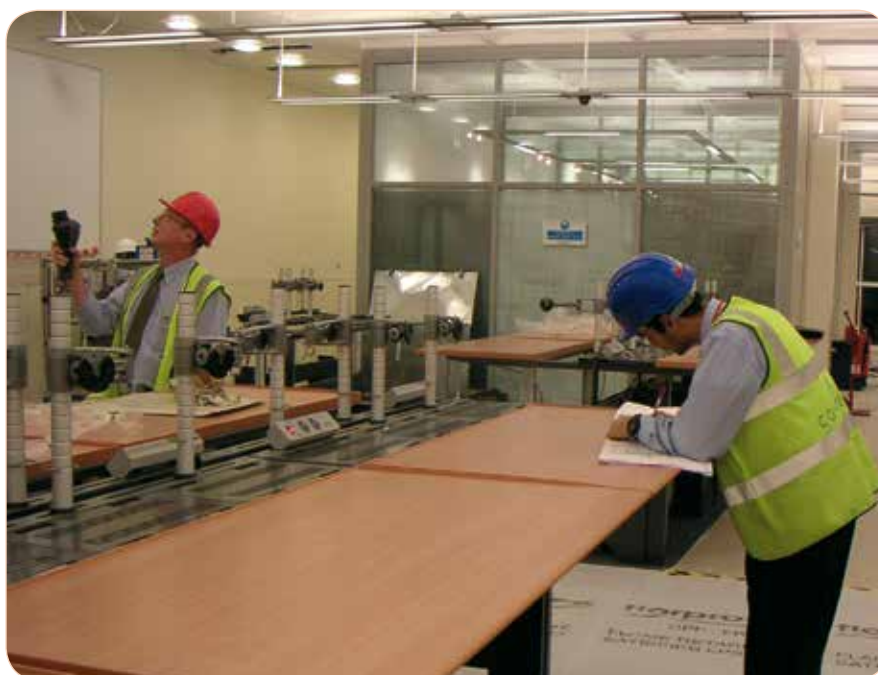
Main image: Commissioning involves a multitude of inspections, assessments and preparations.
