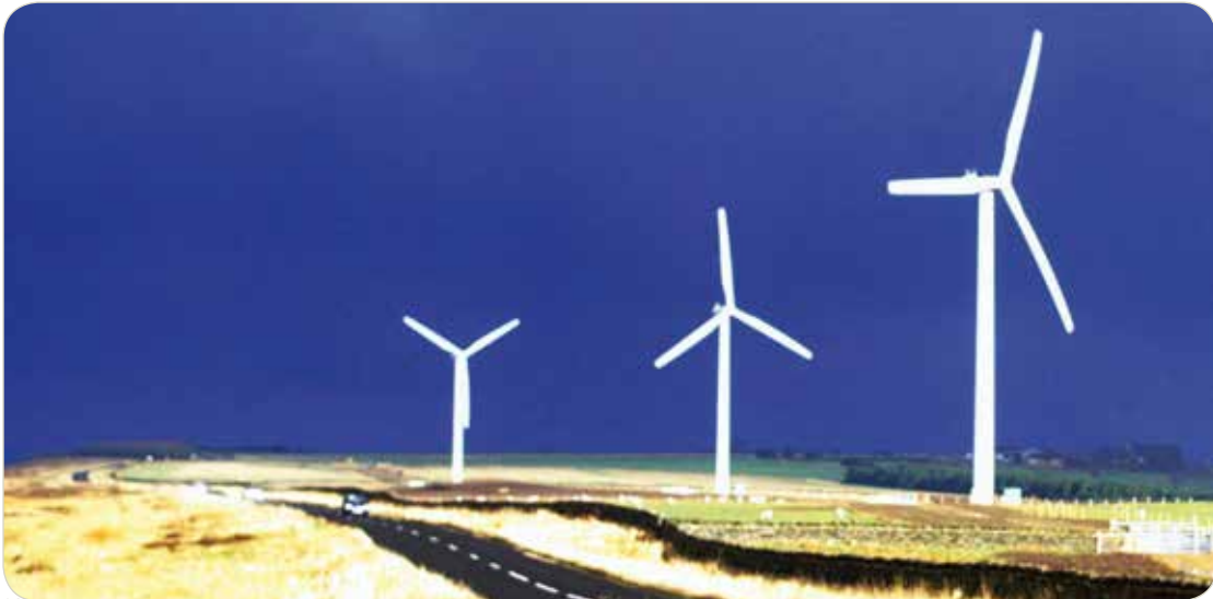
Harnessing the power of nature to provide sustainable energy, the High Hedley Hope wind farm, County Durham, UK. Picture courtesy EDF Energy.
